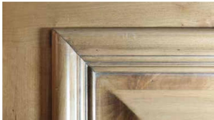
From top: Ogee-Ogee (C5) sticking and panel profiles; Square-Ogee (A5) sticking and panel profiles, with SM4 applied moulding.
